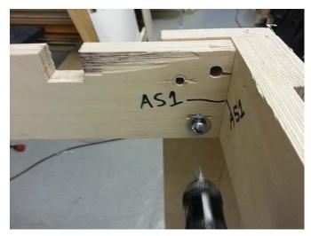
**10.** Place the structures where it should be (normally in the middle of the room). Make sure every sets of legs are levelled and square.
