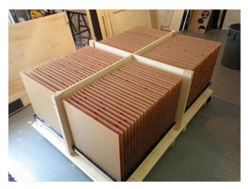
**20.** You now need to lift the LED modules from the crate and install them on the structure. **HINT** : You should turn the LED modules to give a little angle to help to get enough space for lifting. They are identified (A1, A2, B1, B2) so you can find the place they fit on the structure.
